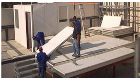
Figure 5.2: Prefabricated panel stacked at the construction site during construction work
