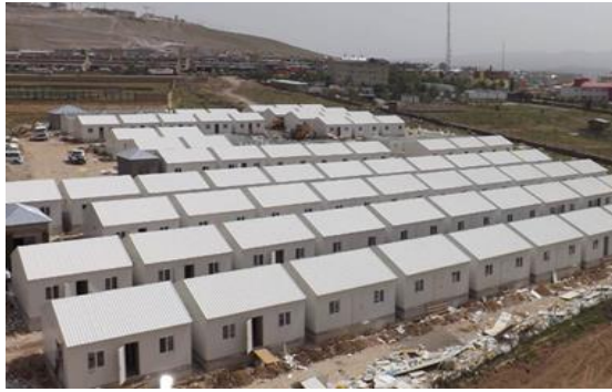
Figure 5.1: Residential layout (mass housing) constructed with prefabricated components
