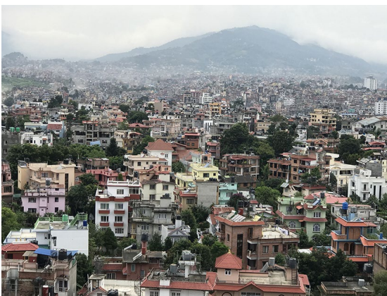
FIGURE 3. In rapidly urbanizing cities of Nepal, such as in the Kathmandu valley, buildings are constructed with no awareness of building codes.
