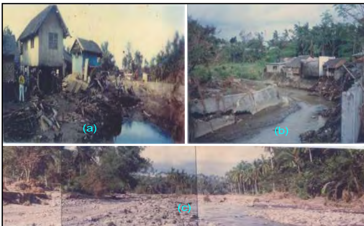
Figure 4-32. (a) Houses destroyed by debris at Malbasag village showing concrete river walls in the centre background; (b) damaged concrete river walls (dike). Note the sharp channel curve at the bridge of Malbasag and Can-adieng. Remains of debris carried by overflowing floodwaters can be seen on top of the concrete wall, and (c) Malbasag River looking upstream at a point where it initially overflowed its bank. The west bank at the left of the photo is heavily damaged as noted by its height. Source: RDCC-OCD 8 (1991).
