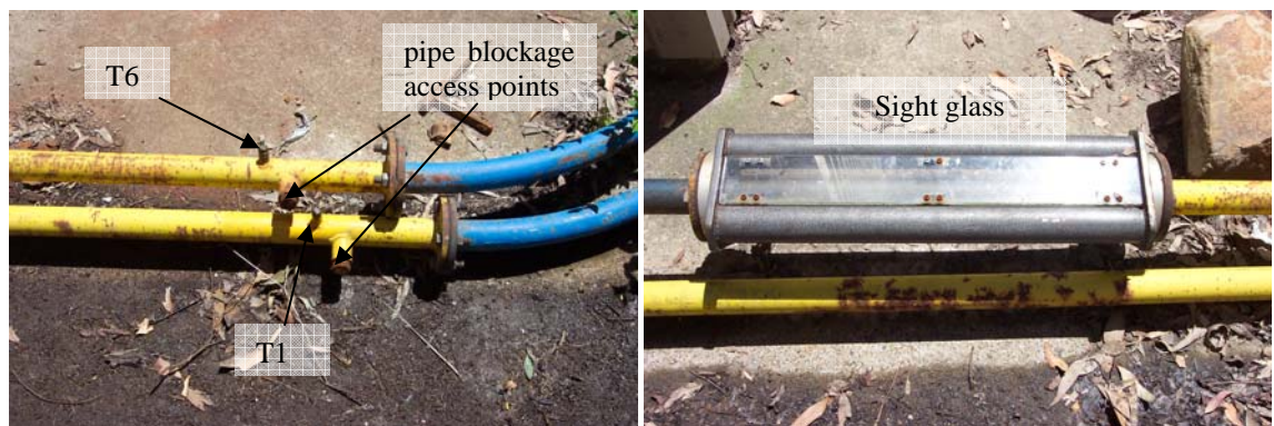
Figure 40, pictures of transducer and pipe blockage access points and sight glass
