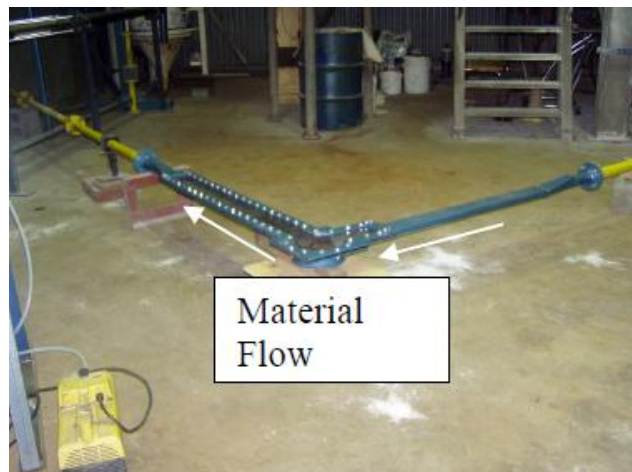
Figure 1-1: The mechanical arrangement from a gas-solid two phase flowing pipeline. (From CIEAM report, 2006) [1].
